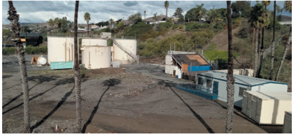
The site has been a fire department training facility since 1991.
