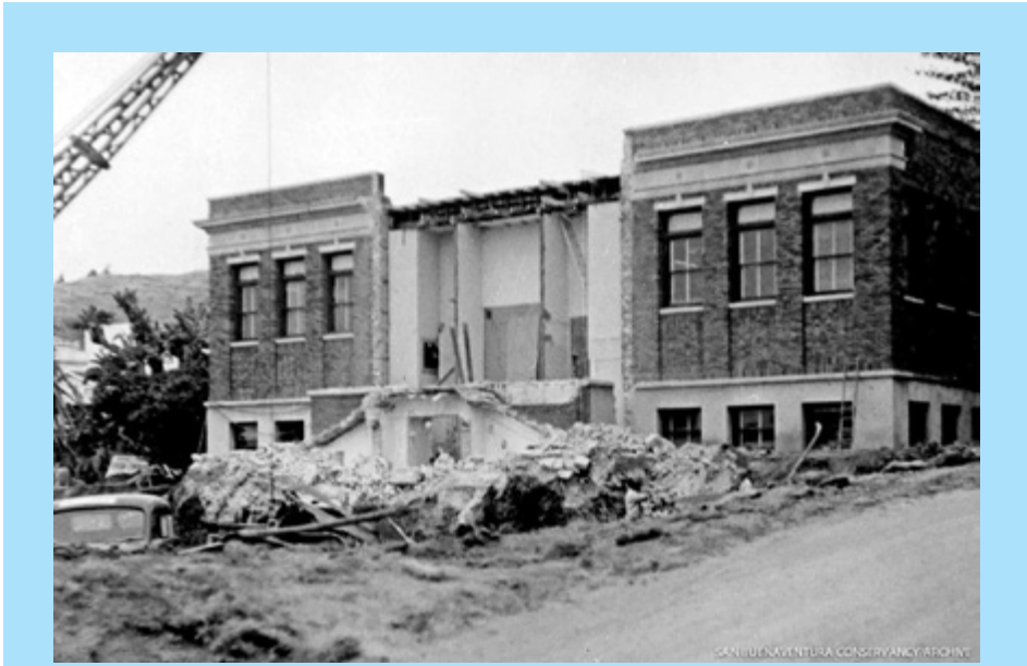
The original E.P. Foster Library on Main St. It is still there located behind the existing library and part of the library.
