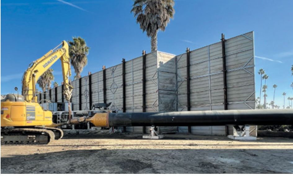
42" diameter pipe was pulled under the Ventura Harbor.
