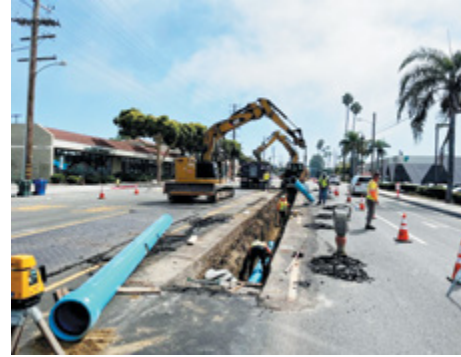
Midtown to Westside Interconnect construction underway on Telegraph Rd.
