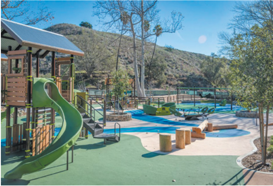
Arroyo Verde Park's main play structure was destroyed in the Thomas Fire.
