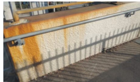
Walkway over the freeway to the pier.
