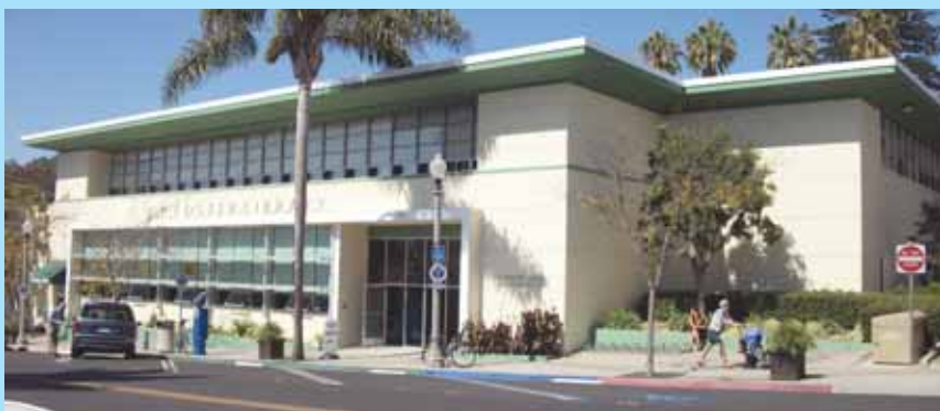
After much discussion and debate, between the library commission and the Historical Preservation Committee about what color to paint the downtown E.P. Foster Library, the library has finally been painted. On May 7th, 2012 the City Council ruled in favor of the paint palate recommended by the Library Advisory Commission. The main building has been painted Parchment, with the trim painted Historical Green and Cream. E. P. Foster Library was built in 1959, and was last painted in 1998.
