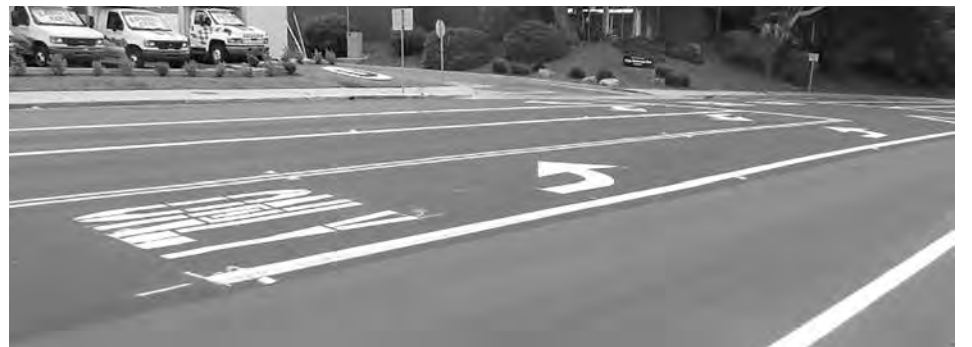
Yet another strange Ventura street condition.
